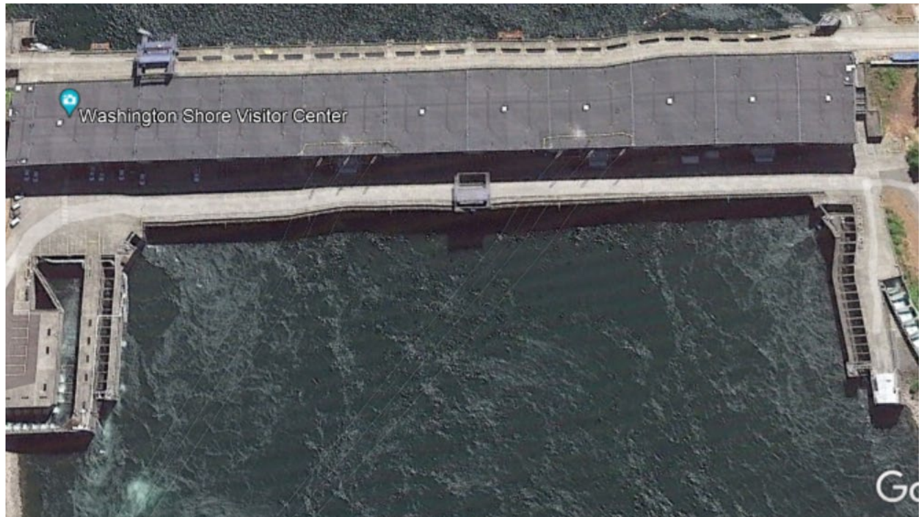
Figure 2 Bonneville Dam PH2. Location of inspection area on downstream side of the structure.
