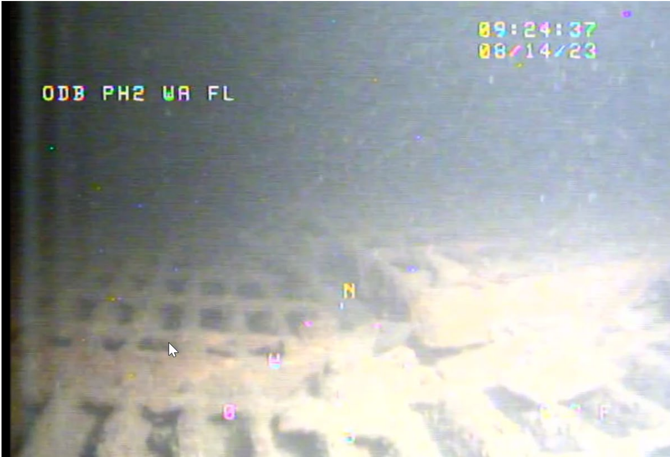
Figure 4. Raised corner grating.
